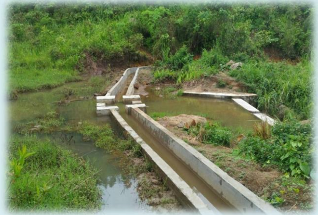
After Construction during Withdrawal and Consolidation Phase
