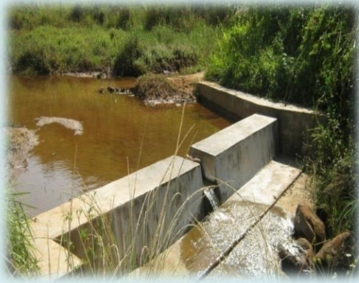
After Construction during 2 nd Year of Project period
